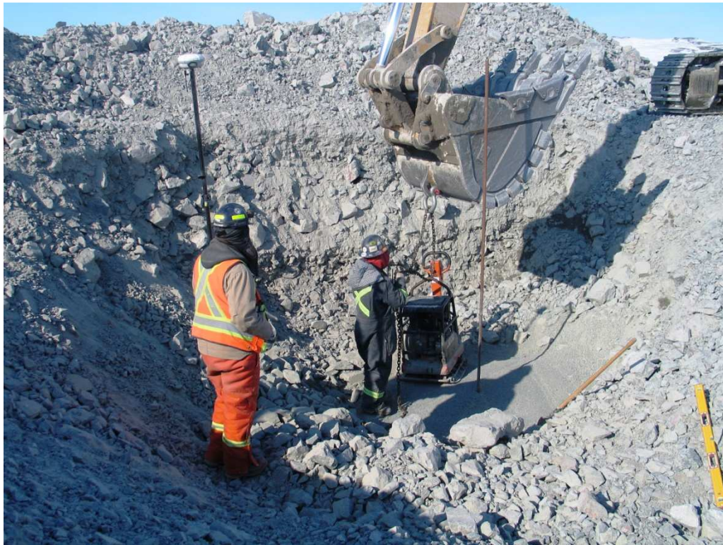
Photo 8: Survey monument is placed, and backfilled with \frac{3}{4} in crush. Small packer has finished packing around the pipe. Surveyor is recording crush. Large excavation was for safety considerations. Packer was moved with chains.
