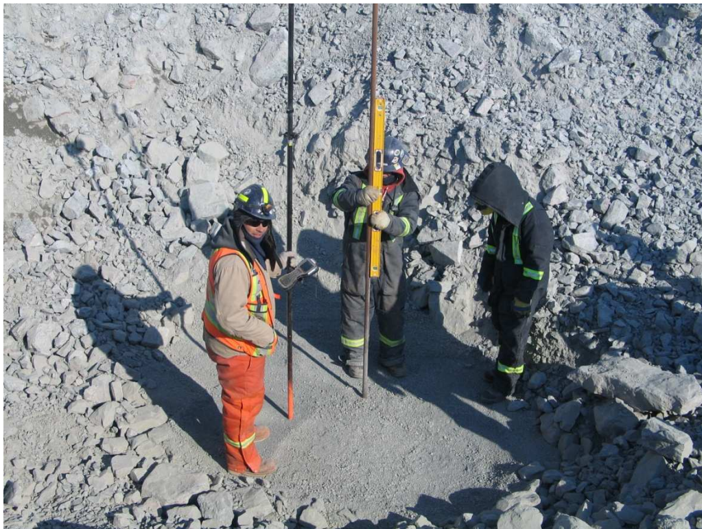
Photo 9: Checking vertical alignment.
