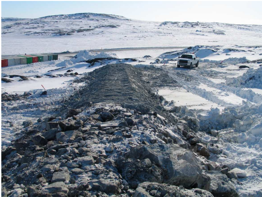
Photo 2: RBTF berm, from top facing east. Some original berm material was used to construct the first section
