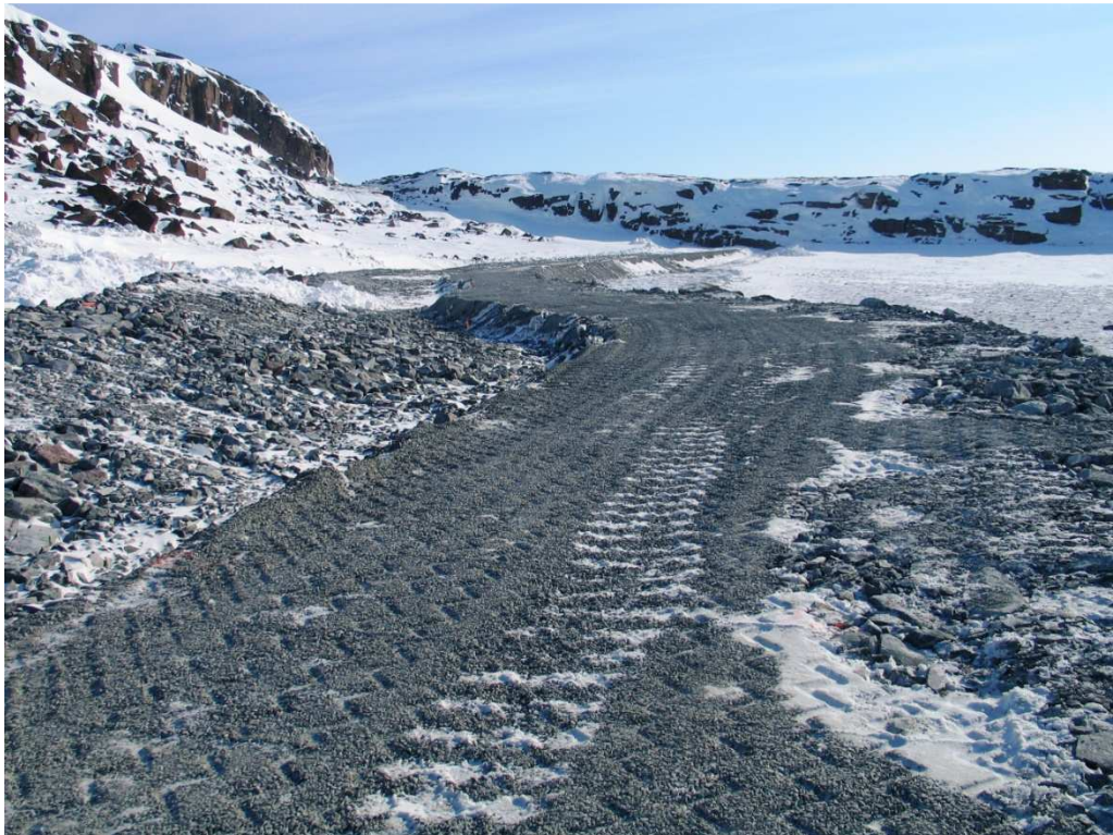
Photo 3: Top of diversion berm Sta 5+00 facing east. Note that crush was placed only to the design width.
